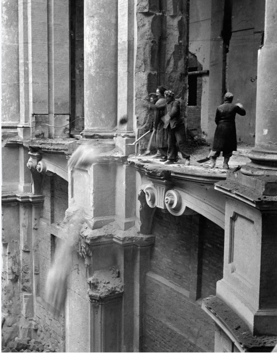
Women work together to clear rubble in these three photographs.
